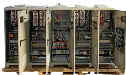
Parallel Configuration with Central Bypass
